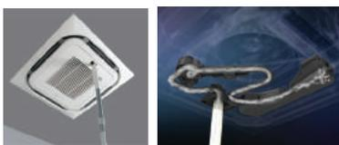
The cassette has an optional self-cleaning filter mechanism to clean the filters daily and prevent increased energy consumption caused by filter loading. The mechanism comes complete with a vacuum cleaner connection to allow for periodic emptying of the collection box.
